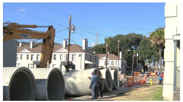
Figure 40. Construction workers dig a massive ditch to accommodate these pipes.
